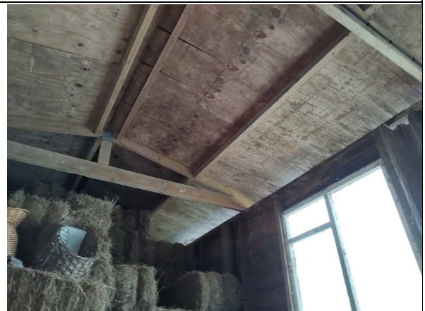
Photograph 6 – View of the internal roof structure with plywood present under the felt and the window on the northern elevation.
