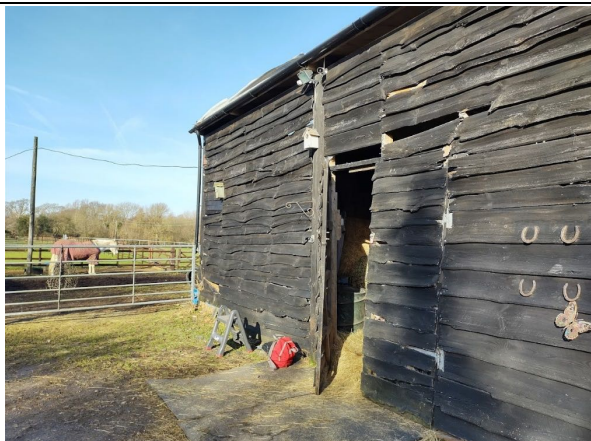
Photograph 5 – Southern elevation of building showing missing sections of weather boarding around existing door.
