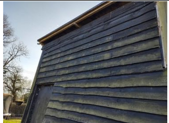
Photograph 4 – Northern elevation of barn showing boarded up door, well-fitting cladding and gaps at the eaves.
