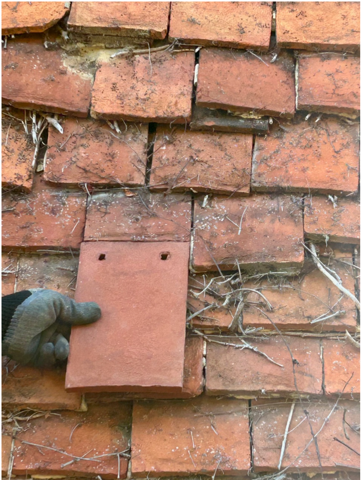
Figure 2 Tudor Sussex Red tile against existing in-situ
