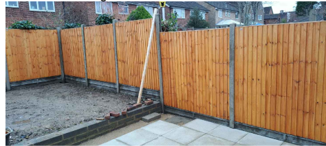
View A - Showing As Built Fence
