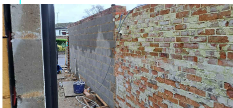
Internal View of Refurbished Wall
