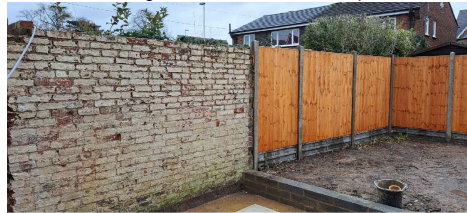
View B - Showing As Built Fence and Wall prior to Cladding
