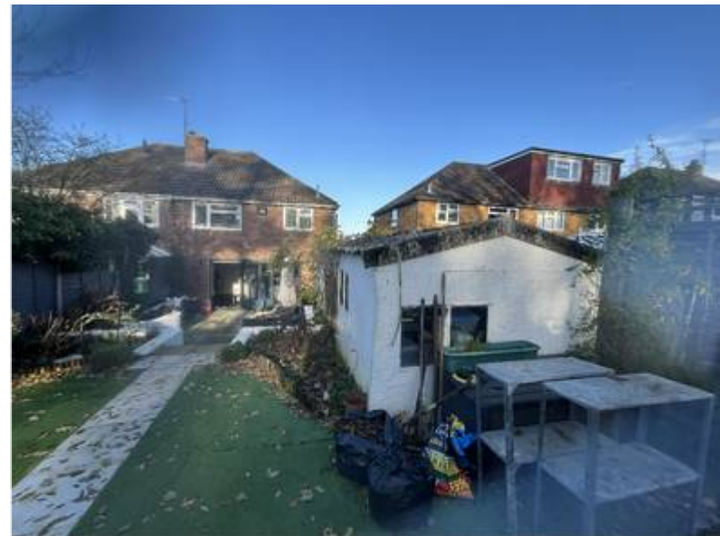
Image 4 - existing garage rear face
