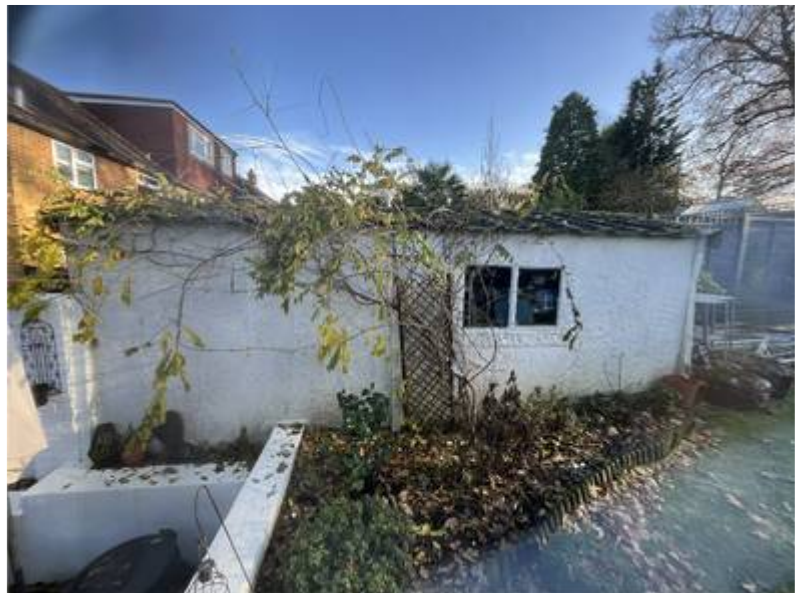
Image 3 - existing garage side face
