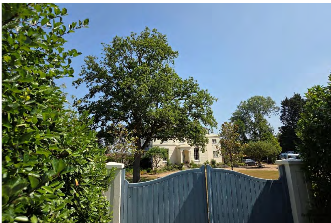
Plate 20. Grade II Listed The Old Rectory from the southwest
