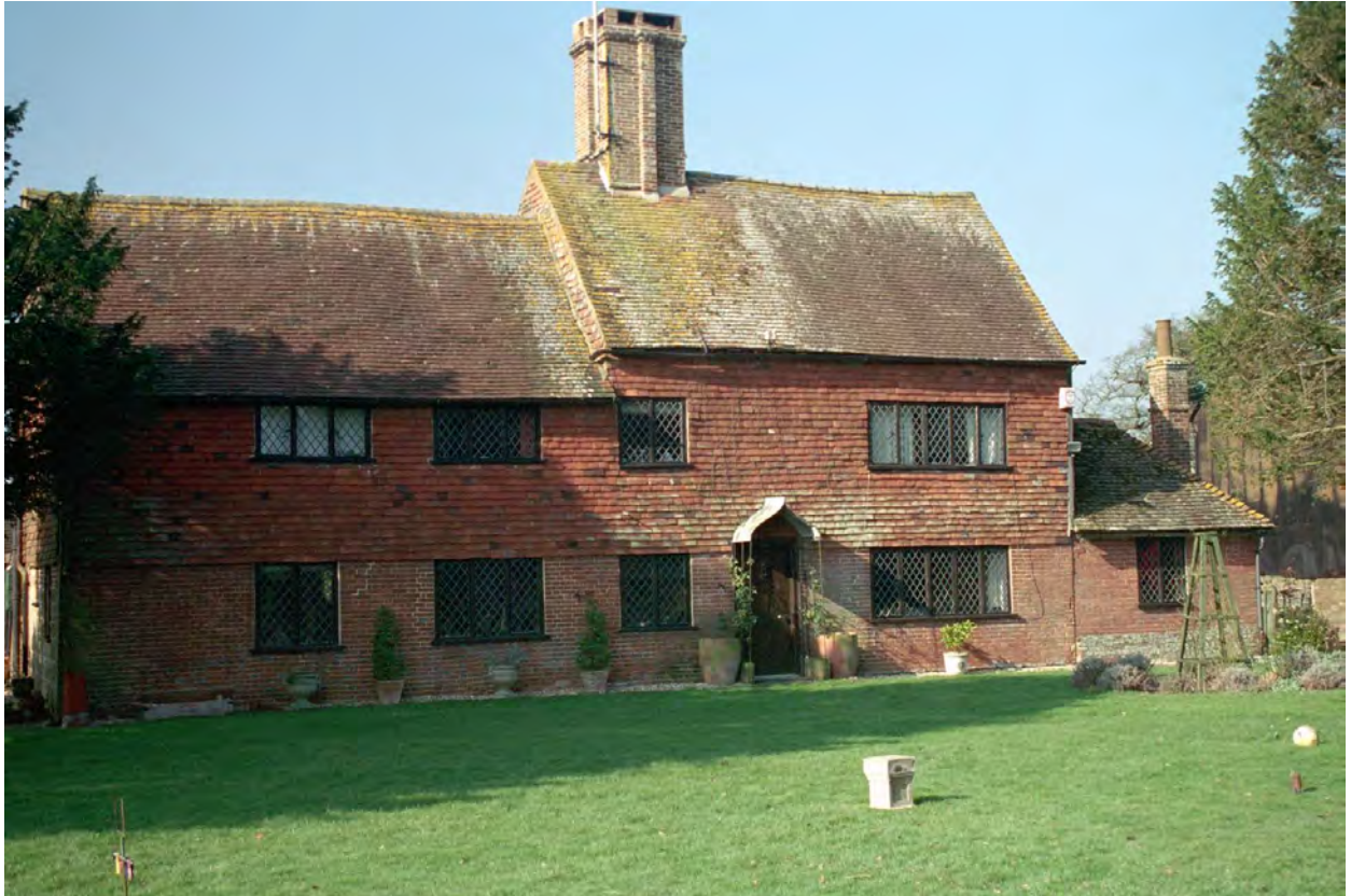
Plate 22. Grade II Listed Park Farmhouse looking west
