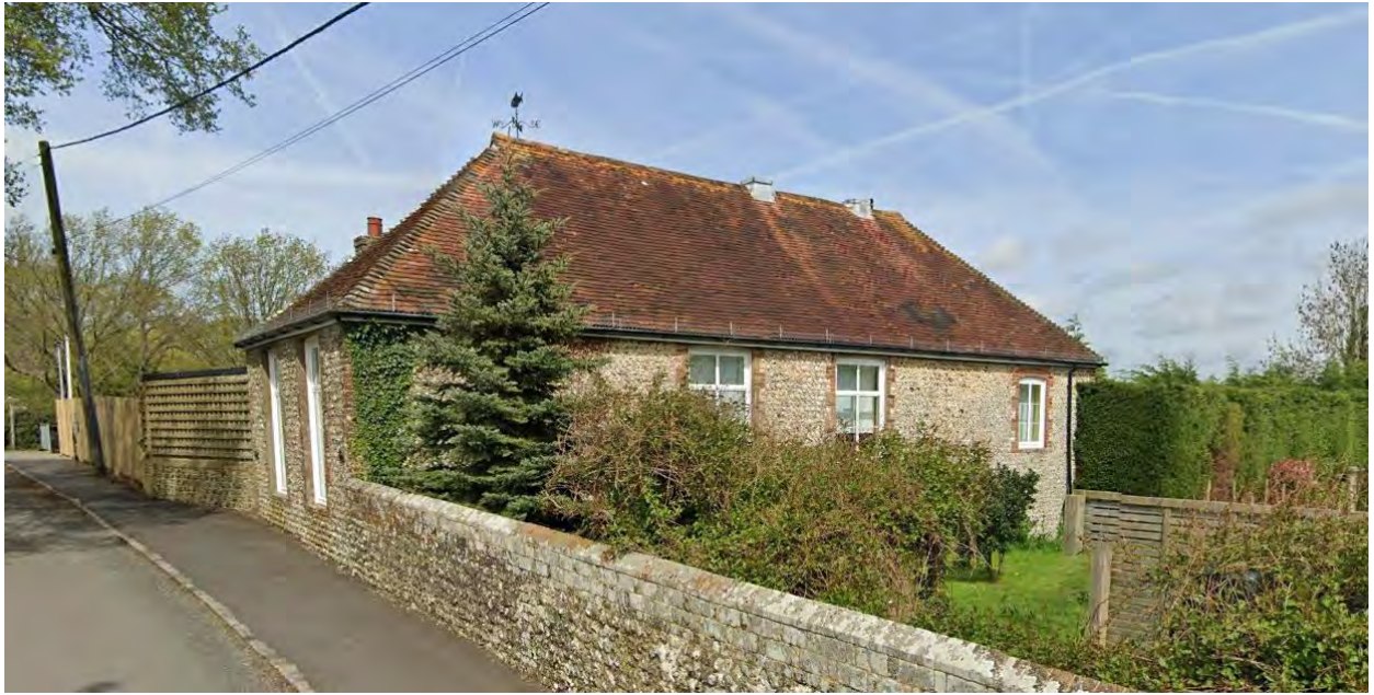
Plate 20. Non-designated School looking northwest (Streetview)
