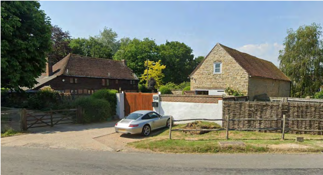
Plate 13a. Curtilage Listed Shepherd's Barn South (left) and Shepherd's Barn North (right), looking south-west © Streetview
