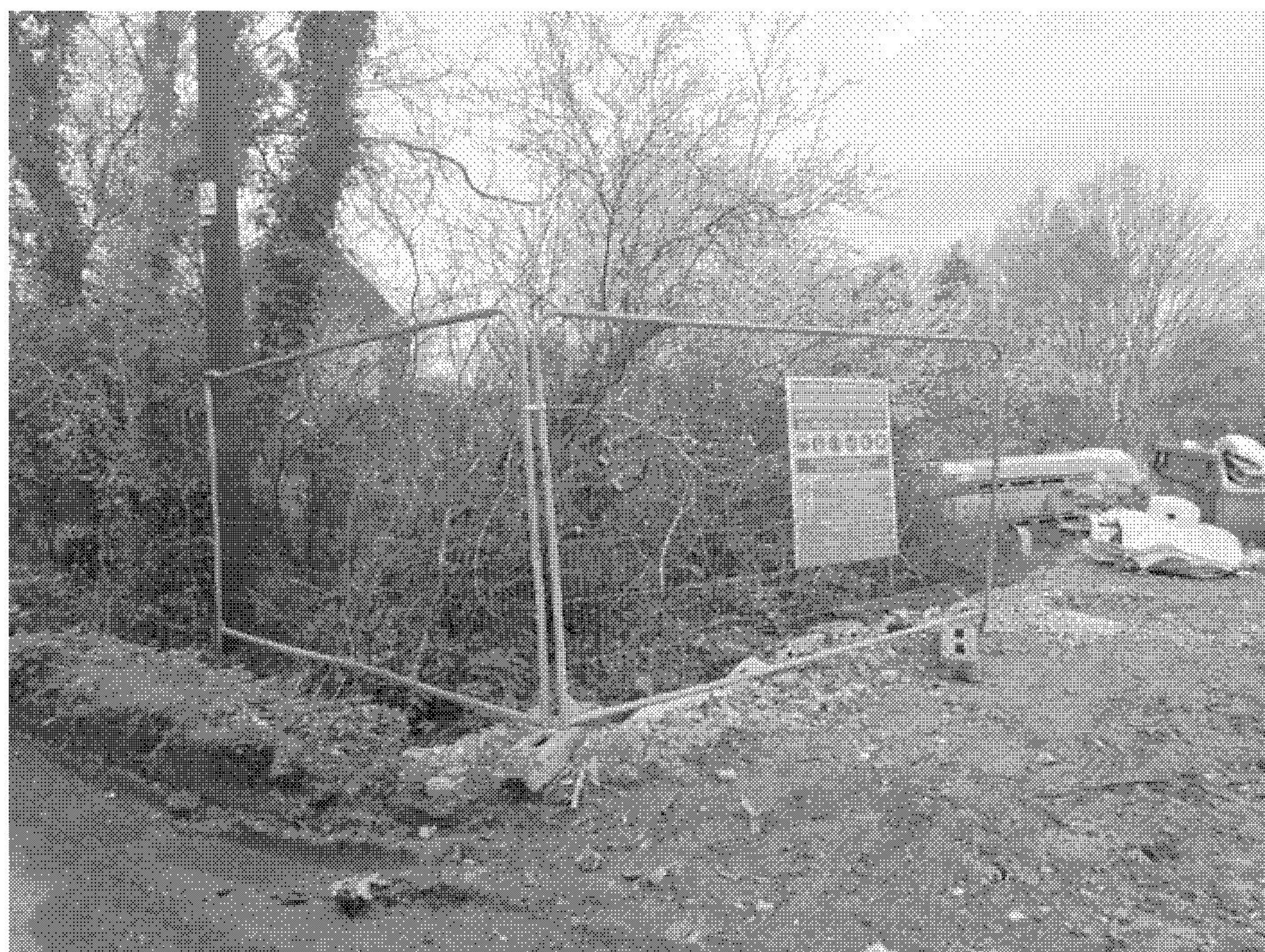
Image 16 A gap in H14 with a storage and facilities area at the rear.
