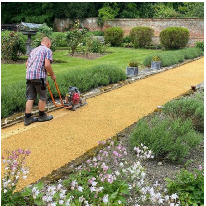
Hoggin self binding gravel footpath
