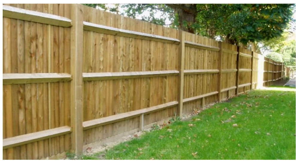
Close boarded timber fencing to boundary, 1.6m height
