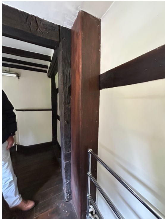
Figure 4 soil stack in bathroom below
