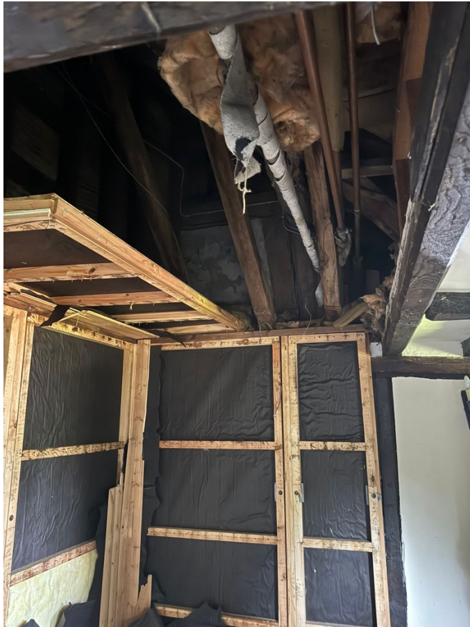
Figure 8 sauna removed and framed lining in progress of removal revealing roof void and missing ceiling joists
