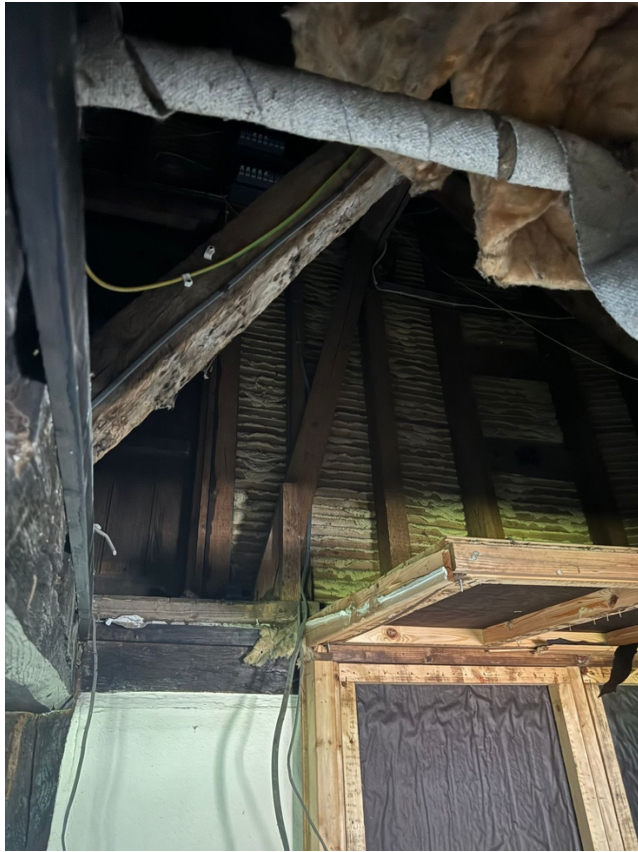
Figure 10 void in loft from sauna removal – note mortices for floor joists in beam
