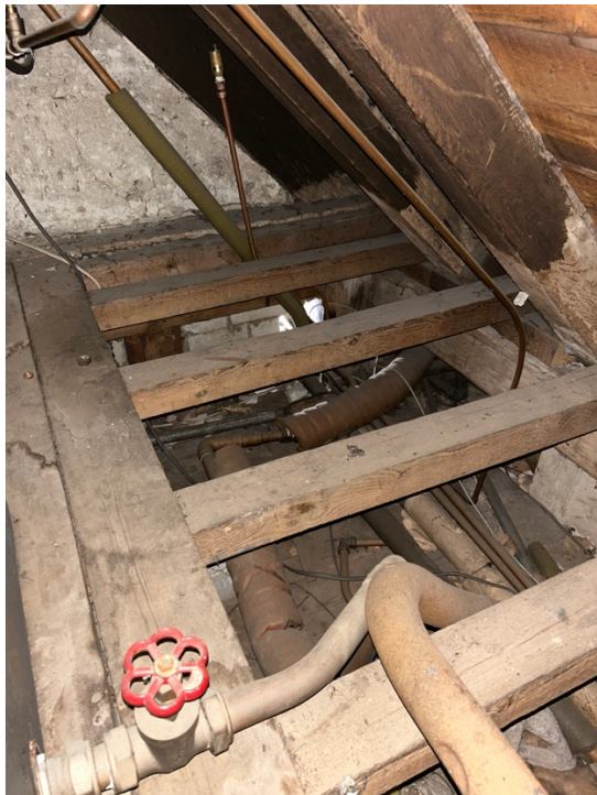
Figure 3 attic void to rear of partition showing opening
