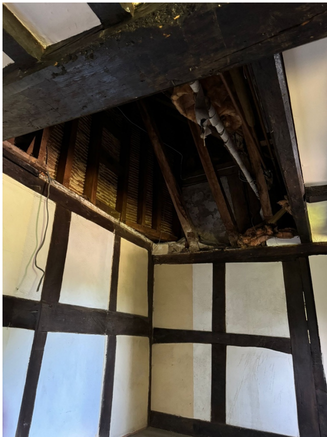
Figure 9 sauna frame removed revealing wall frame
