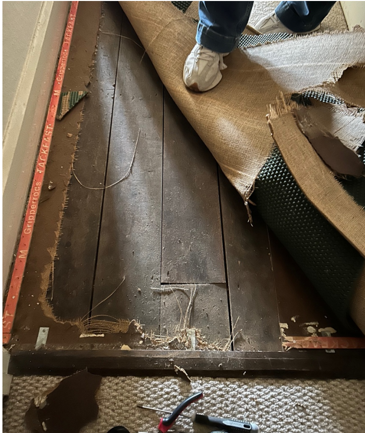
Figure 6 circa C20th machine sawn regular t&g boards in attic room fixed with nails
