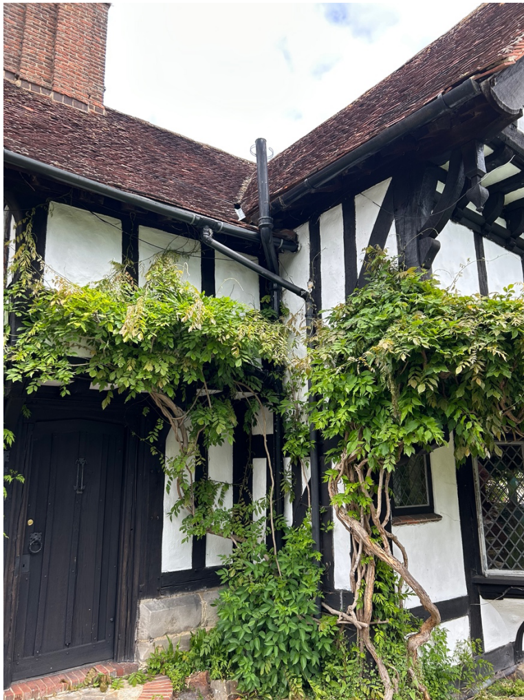
Figure 5 external soil vent pipe
