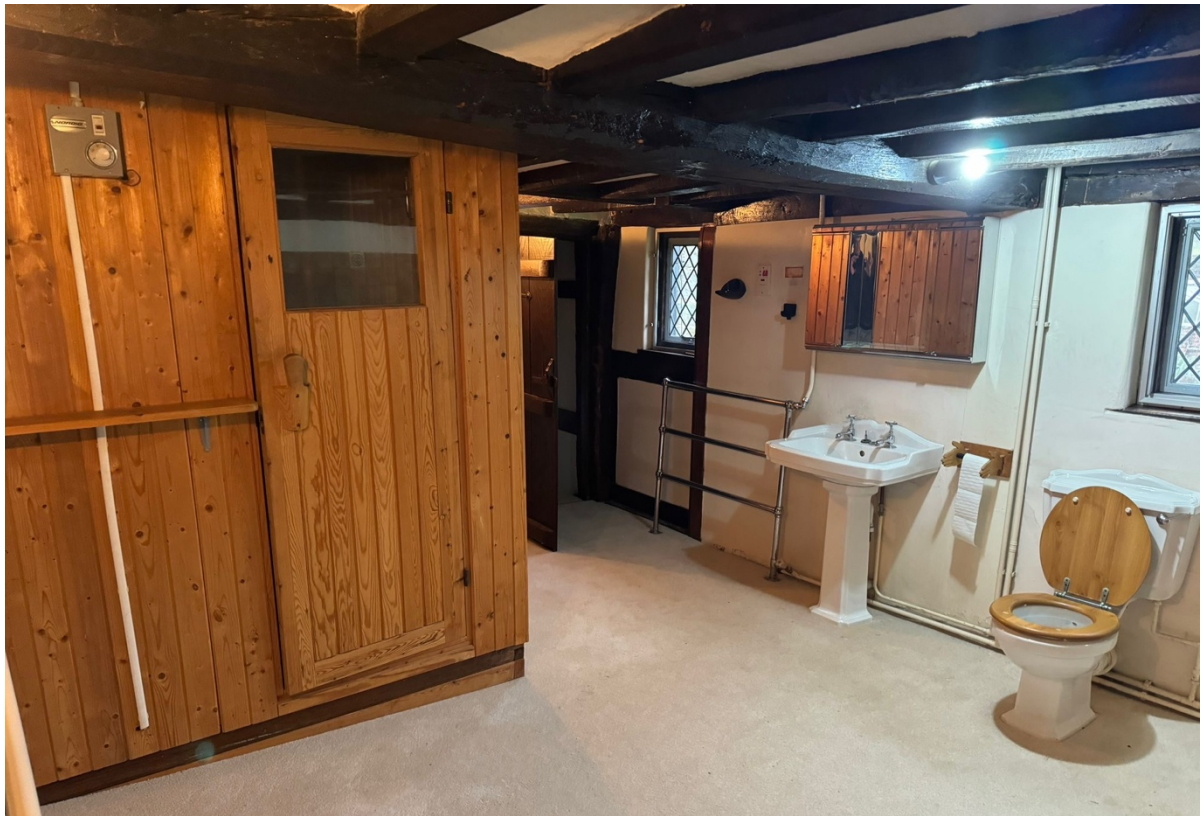
Figure 7 sauna before removal
