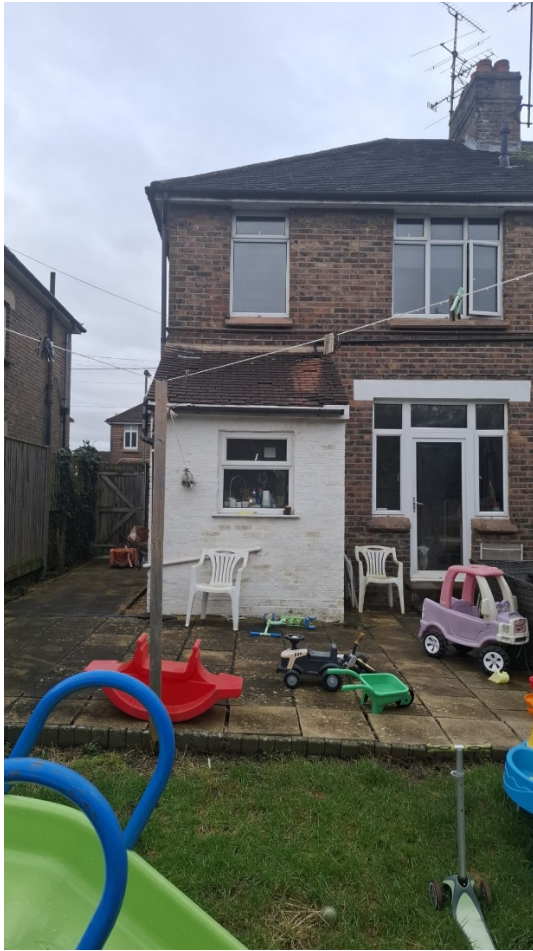
Figure 1 – Photo of existing rear of the property. Side access gate is visible on the left of the photo.
