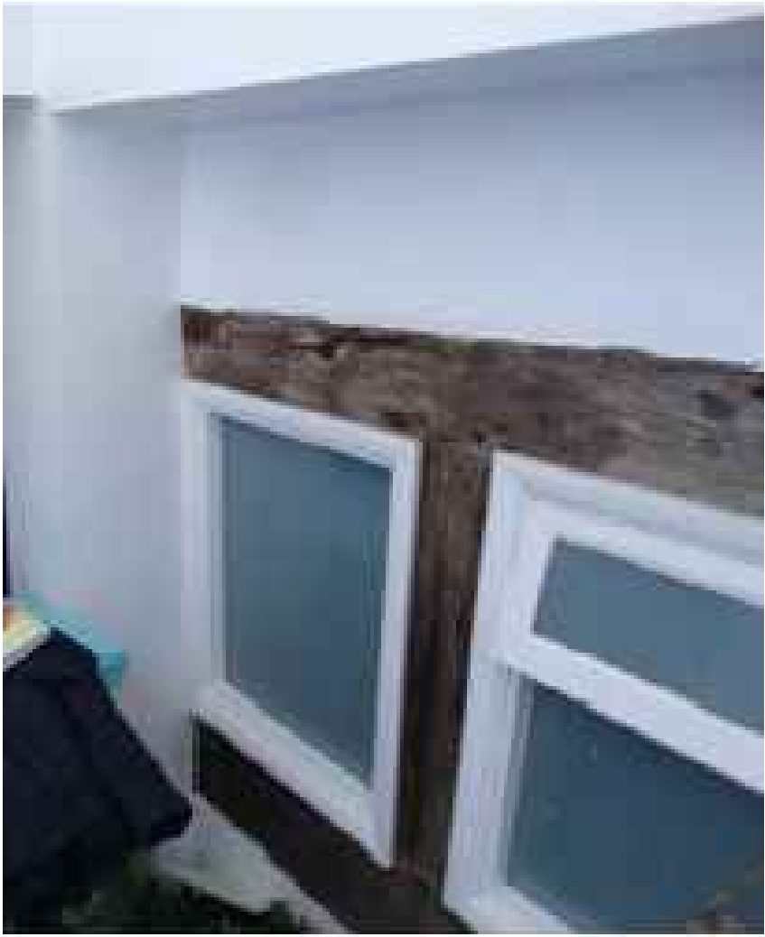
Before: uPVC casement windows before removal
