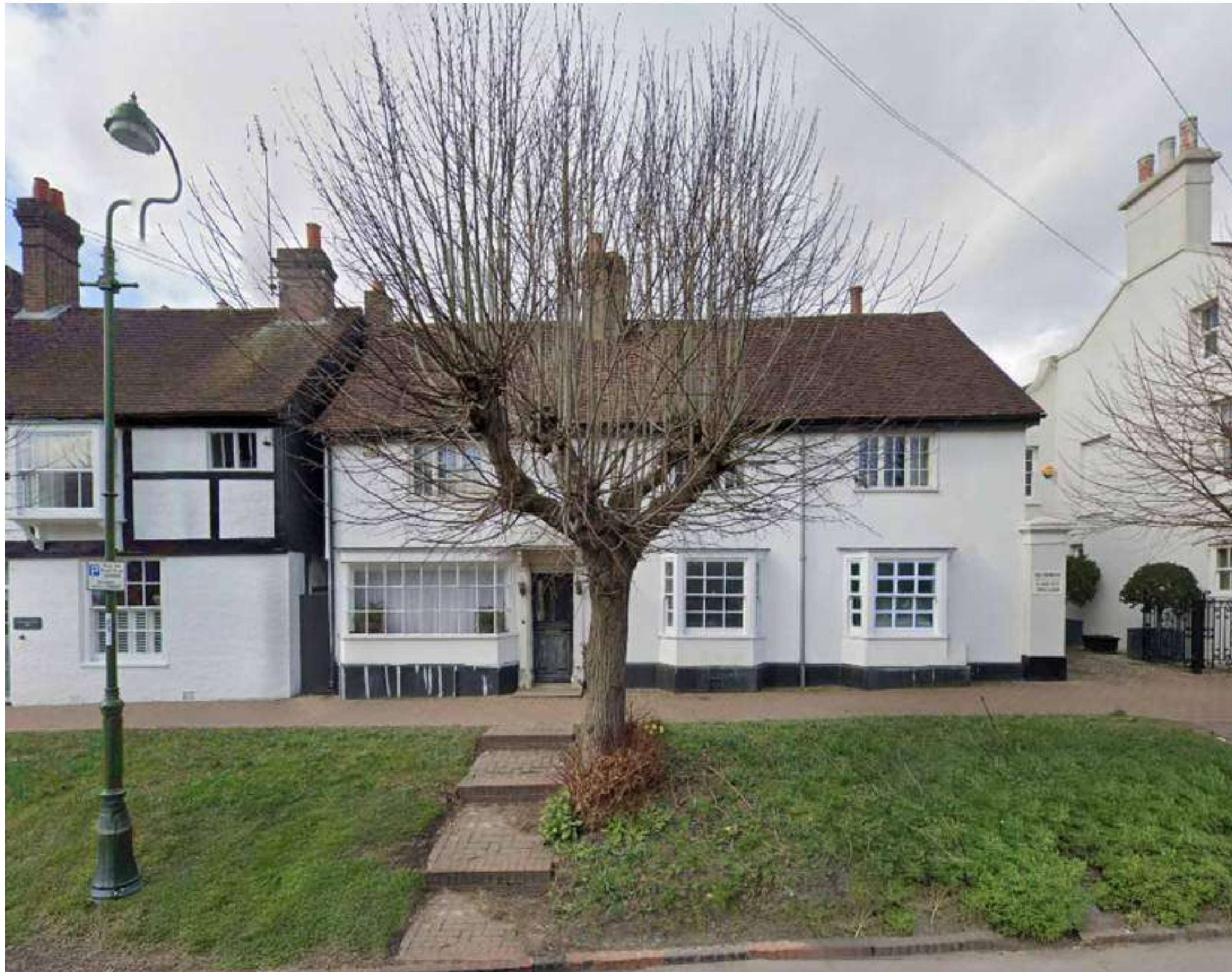
Street view of the facade.
