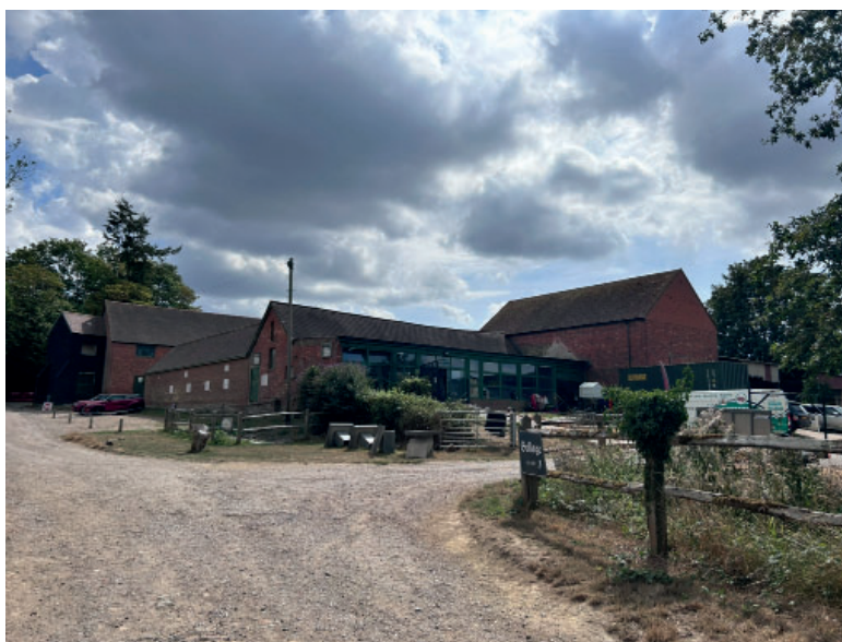
Fig. 12. Imberhorne Farm group as seen from the bridleway looking approximately east (farmhouse screened by trees and built form)
