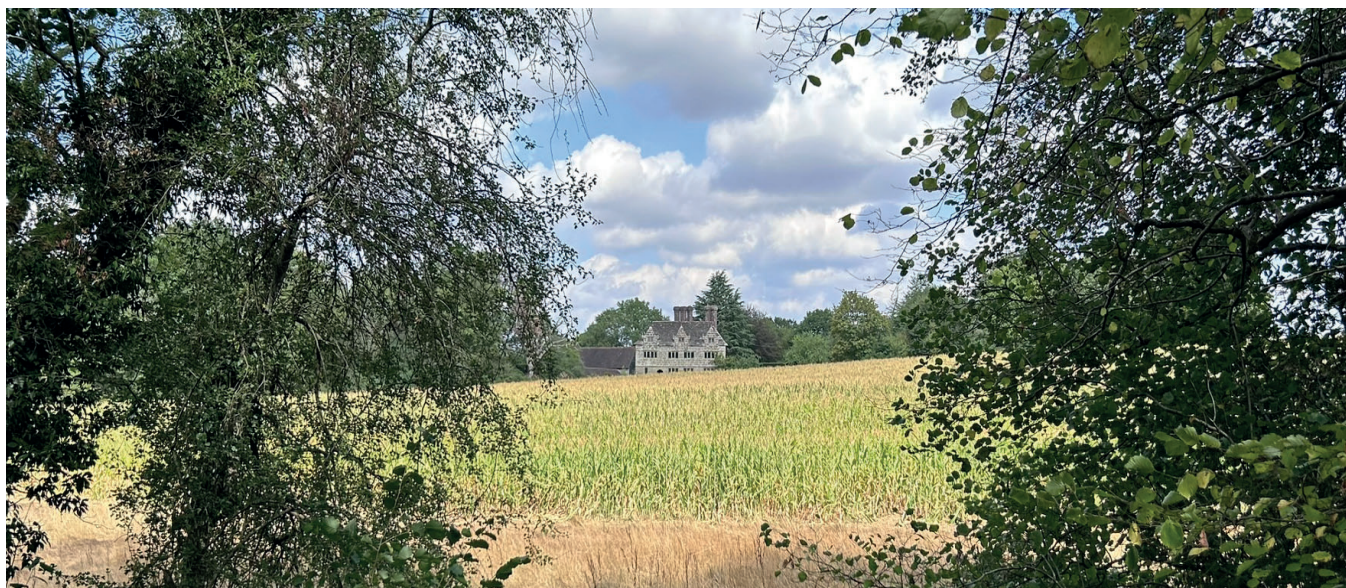
Fig. 13. Gullege south elevation as viewed from Worth Way PROW
