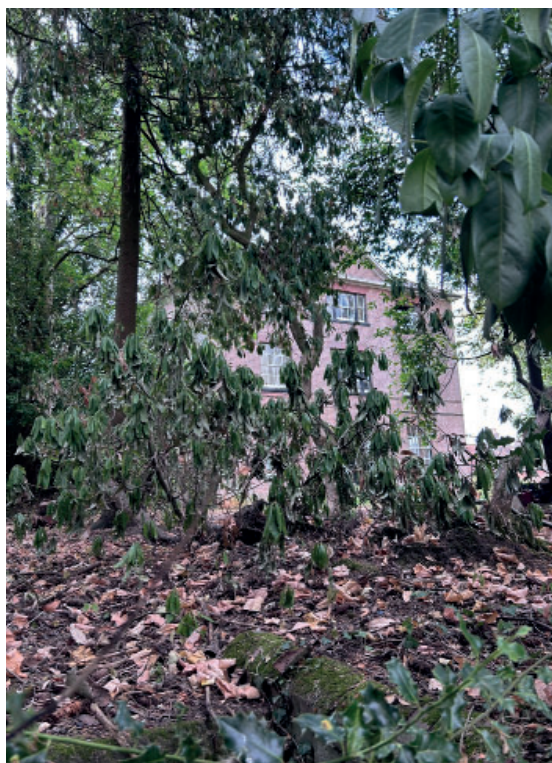
Fig. 11. View to front (south) elevation of Imberhorne Farmhouse from the bridleway
