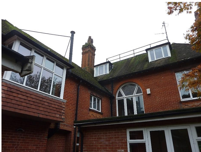
Fig. 4 – The rear of the house, viewed from the south-west, showing pitched roofed section with hanging tiles beneath dormer window, to left, as well as flat-roofed single-storey extension, dormer windows in main roof, with railings to flat roof above
