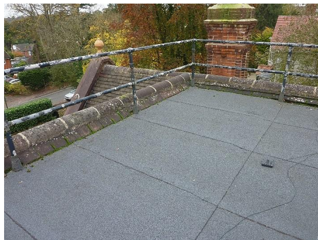
Fig.13 – Flat, felted roof of main house
