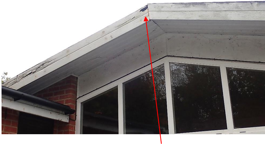
Fig. 9 – Damaged fascia to swimming pool extension
