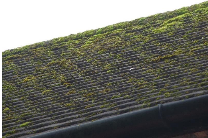
Fig. 6 – Mossy and tight-fitting roof tiles on main house
