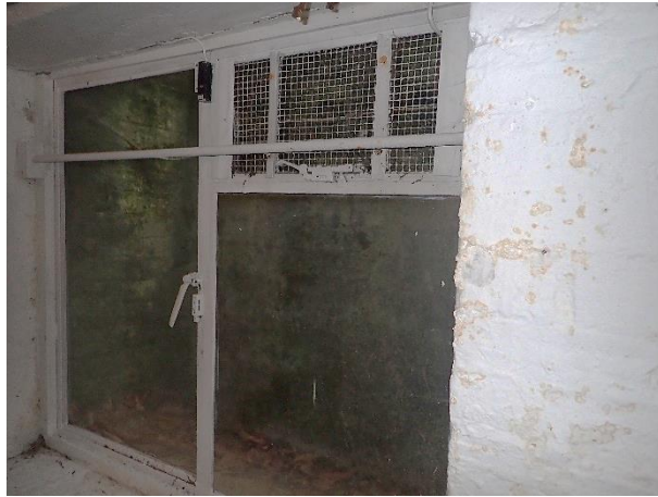
Fig. 15 – Basement window, with meshed section
