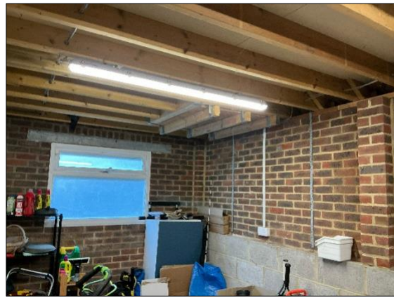
Photograph 8. Garage roof void
