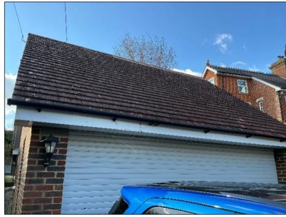
Photograph 6. Eastern elevation of the garage
