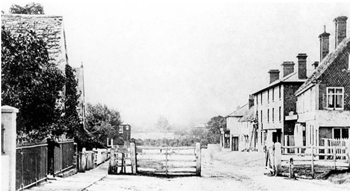
Figure 7-5 – The Toll House with fence and gate looking South down the street
