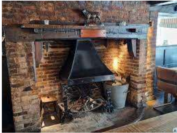
Figure 7-27 – Example of Fire Canopy
