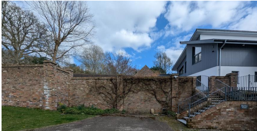
Fig. 5: View from the access track looking east; main house on right
