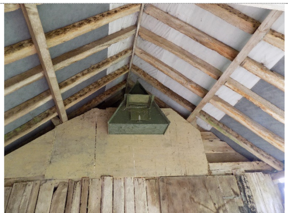
Figure 43: View of the roof structure showing the use of breathable membrane and an owl box located within the barn.
