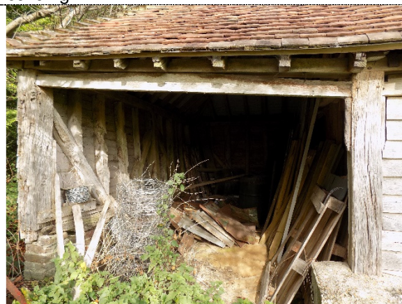
Figure 42: View of the western room
