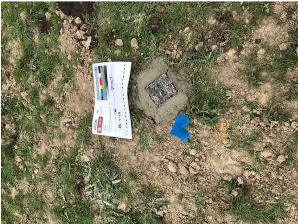
WS116: Post drilling
