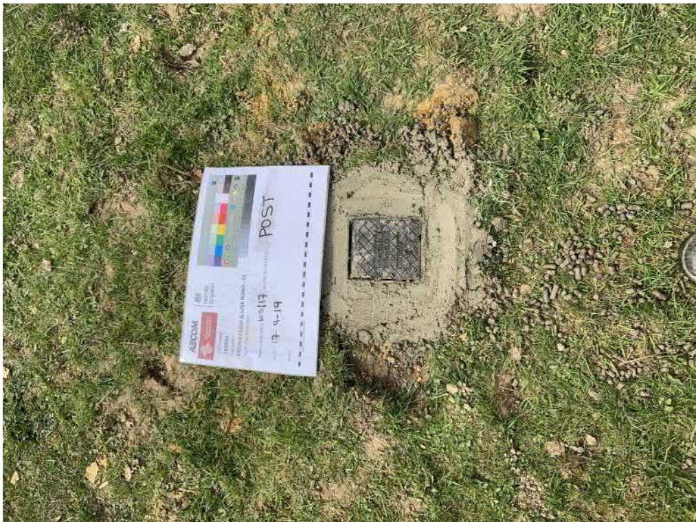
WS117: Post drilling
