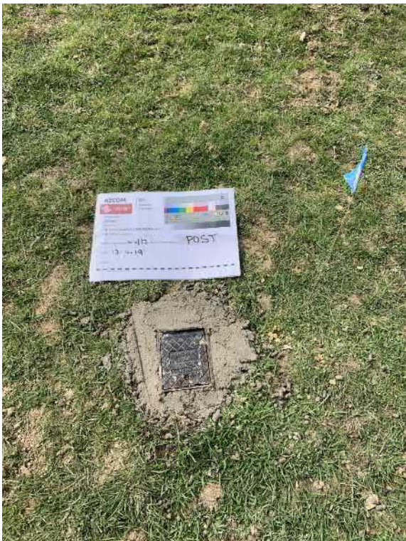
WS112: Post drilling
