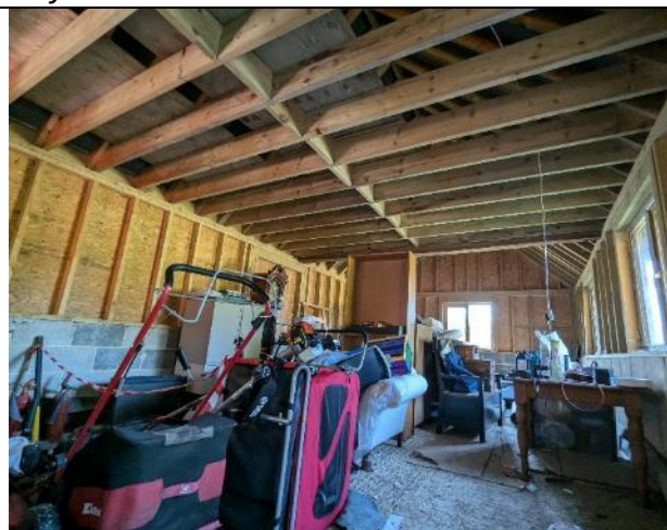
Photograph 8: Internal ground floor of the north wing.
