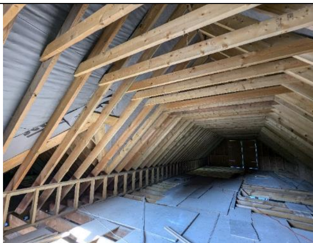
Photograph 7: Internal 1 st floor of the east wing.
