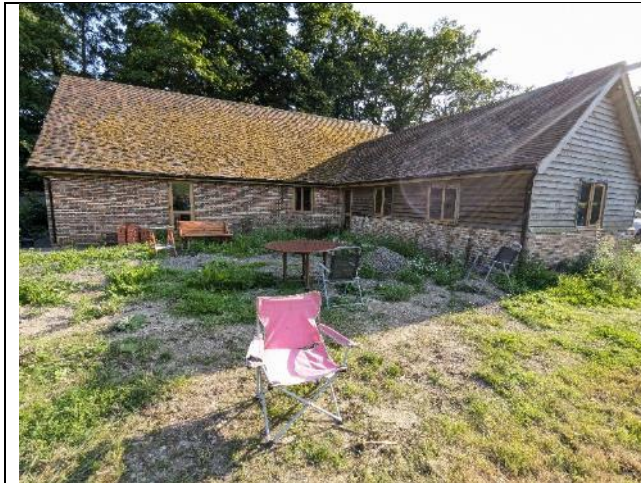
Photograph 1: North and east wings of the barn.
