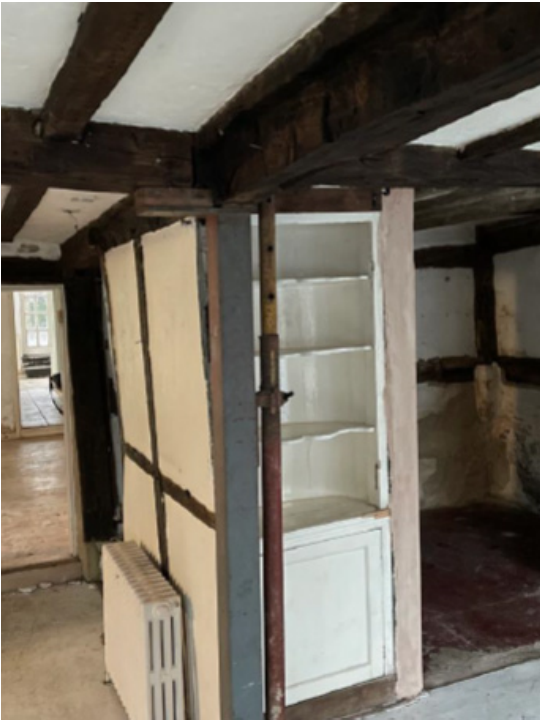
Pre-construction photograph - steel post supporting timber frame
