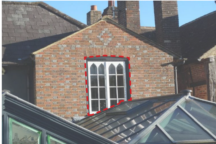
Pre-construction photograph - Victorian window, view from bedroom
