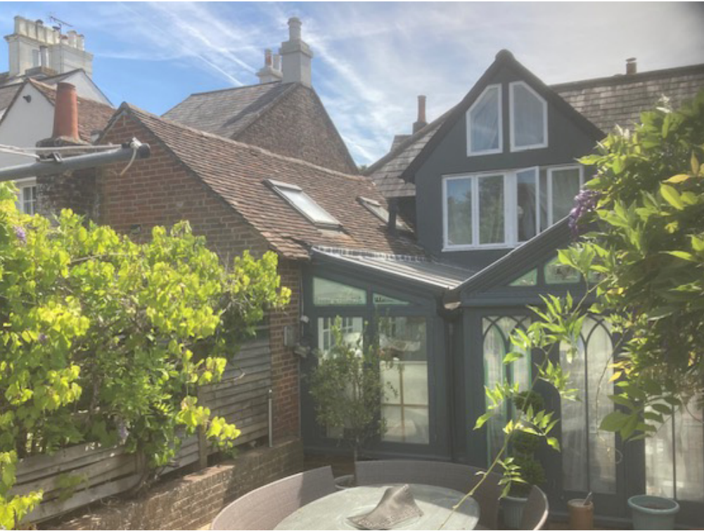
Rear view of Marlow House before works
