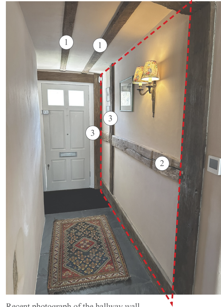
Recent photograph of the hallway wall
