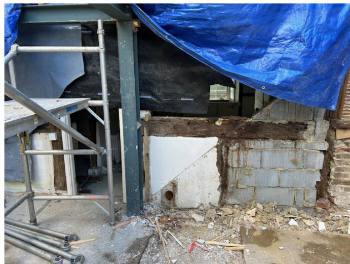
Breeze block within external and internal walls
