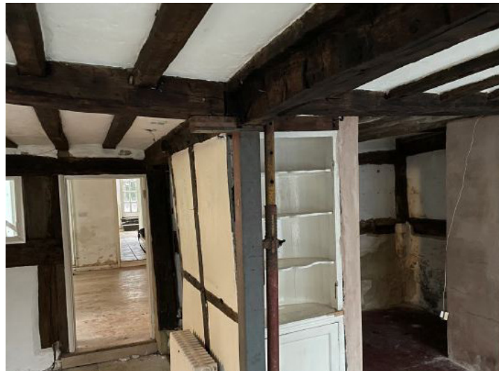
Internal wall and steel beam before removal
