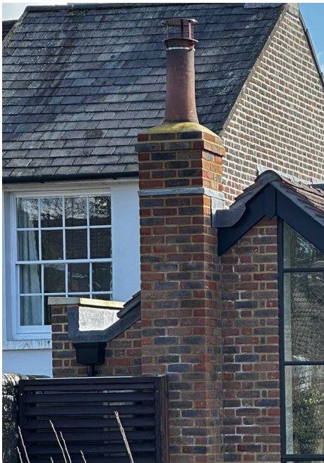
Recent photograph of parapet wall detail
