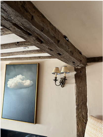
Evidence in the oak frame overhead that there used to be a lateral partition in the current study room
