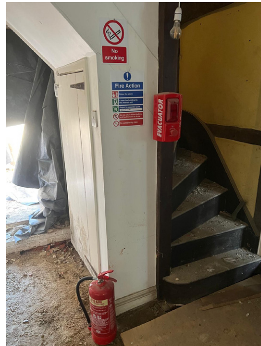
Staircase during demolition works
