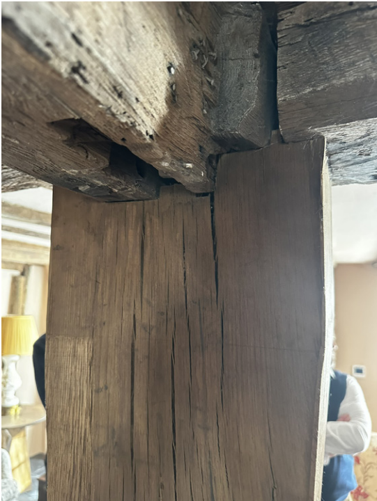
Junction of the traditional gunstock post in seasoned oak to existing ceiling beams
