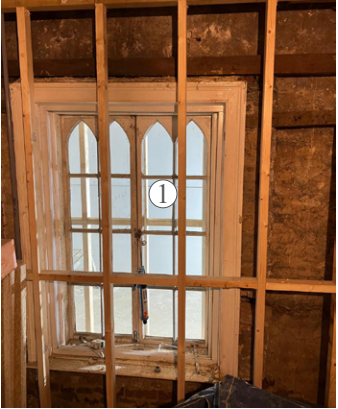
Photograph of the gothic window retained but hidden behind internal wall (wall under construction)
