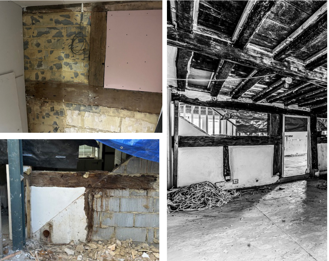
Photographs of historic oak frame prior to restoration
