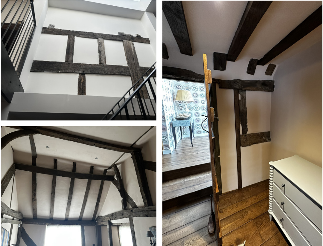
Photographs of restored historic oak frame
