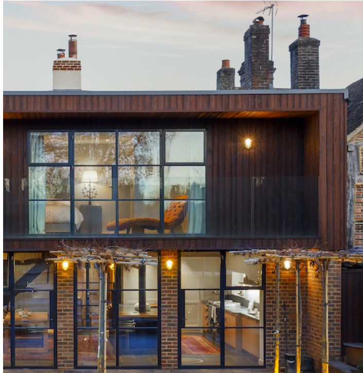
Recent photograph showing mass of historic outrigger visible through glazed openings
