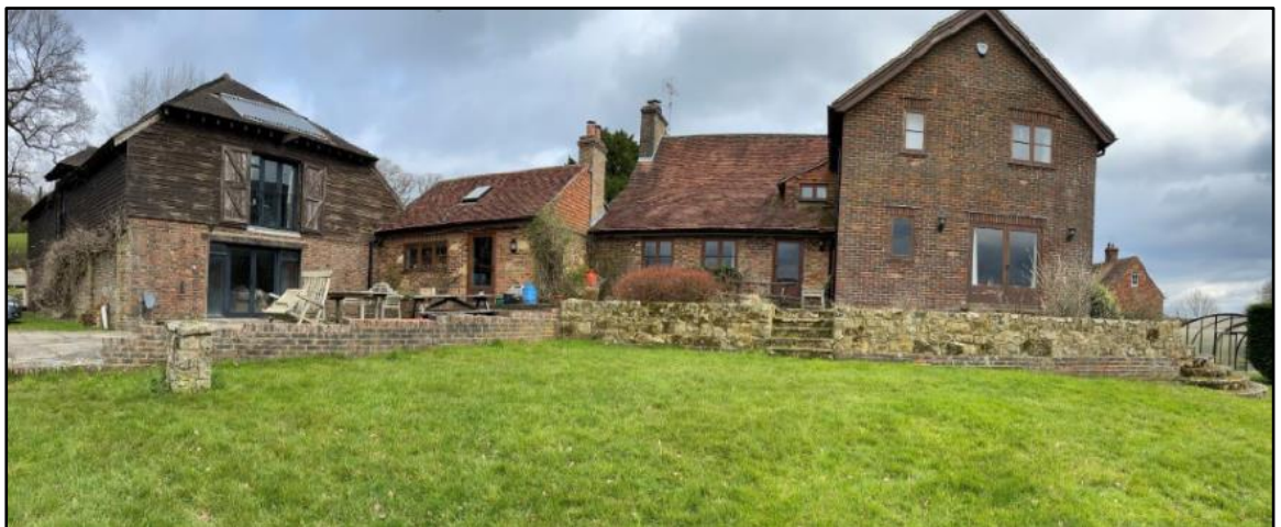
Above – Farmhouse western elevation, with converted barn to the left
