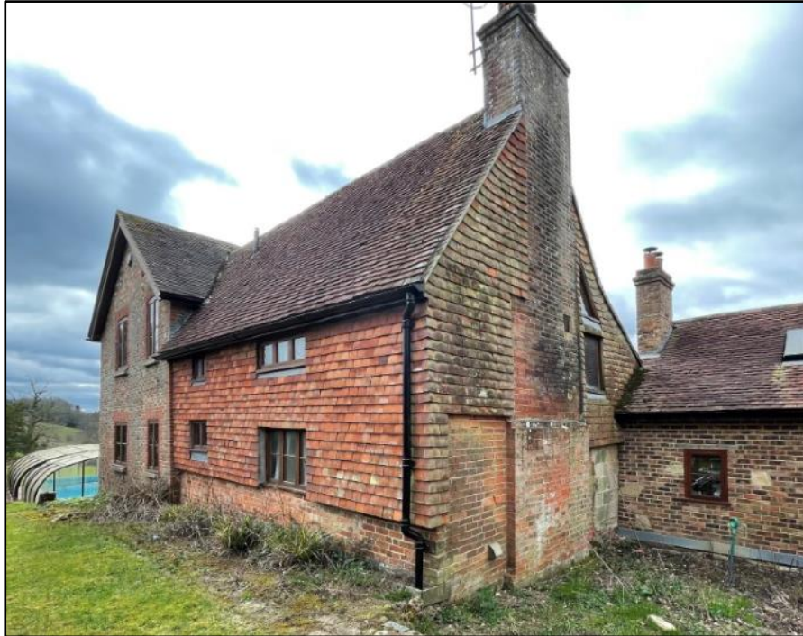
Above – Farmhouse east and north elevation
