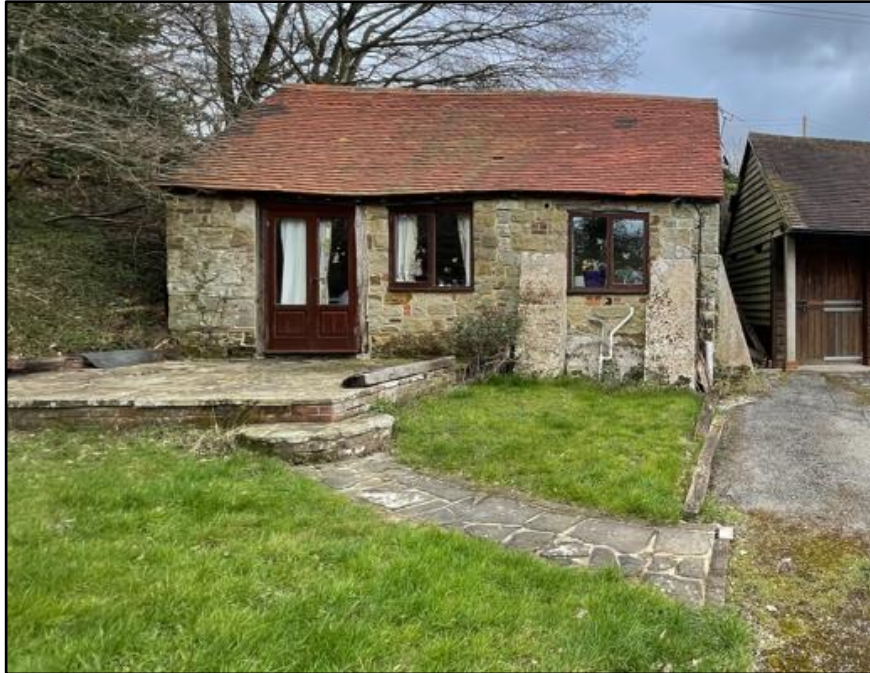
Above – Existing Bothy with front patio where the extension is proposed
