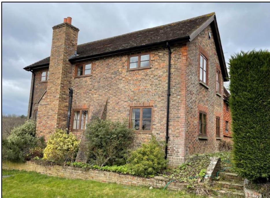
Above – original farmhouse from south
