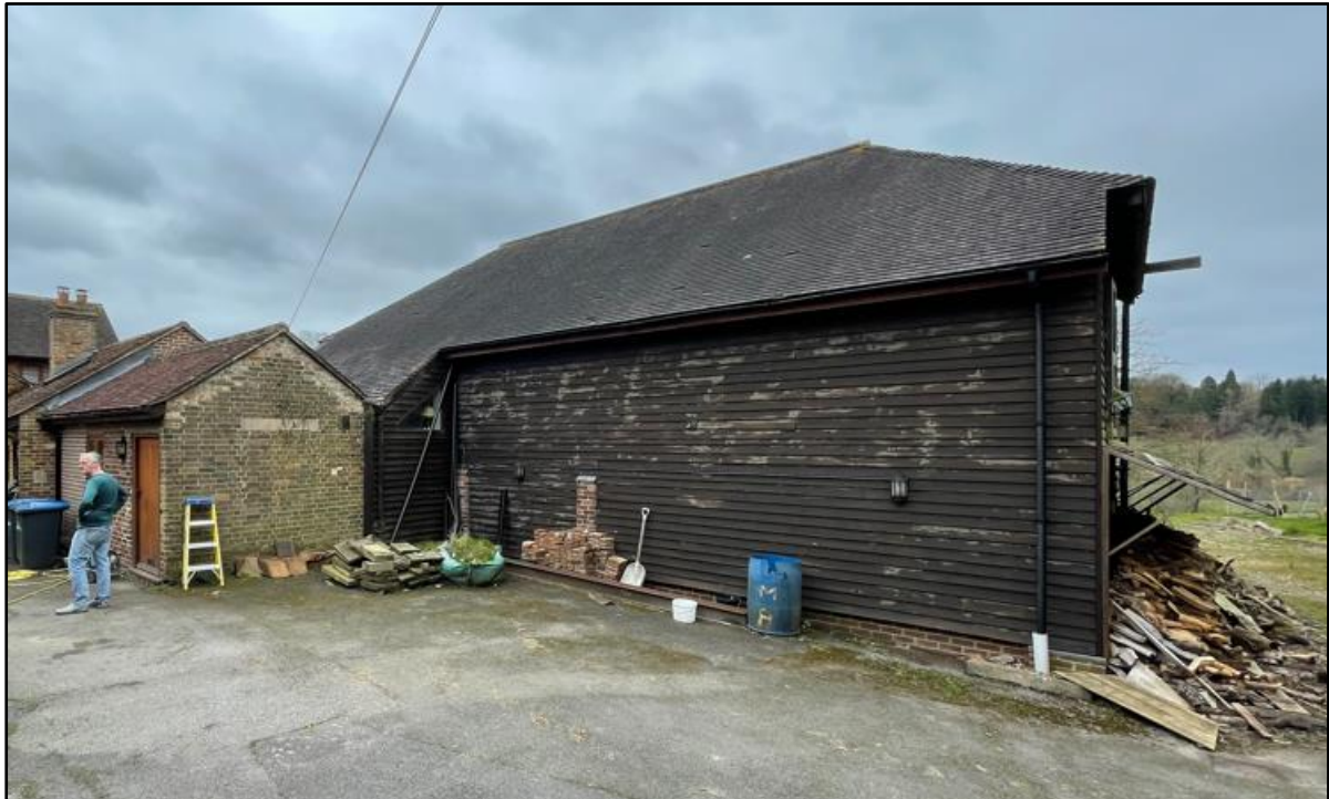
Photo of location of proposed extension to the barn
