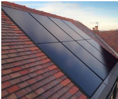
Fig 3.1 Image of Marley Solar tile recessed installation
