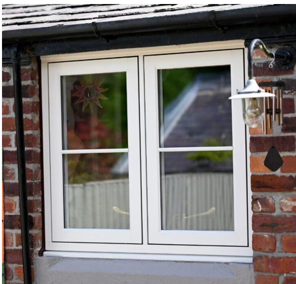
Fig 1.1 Image of Residence R9 flush casement with central glazing bar
