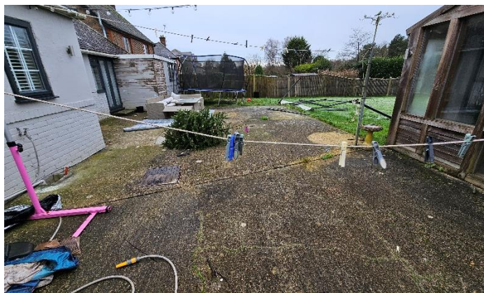
Figure 4. The concrete patio in the rear garden of the property.
