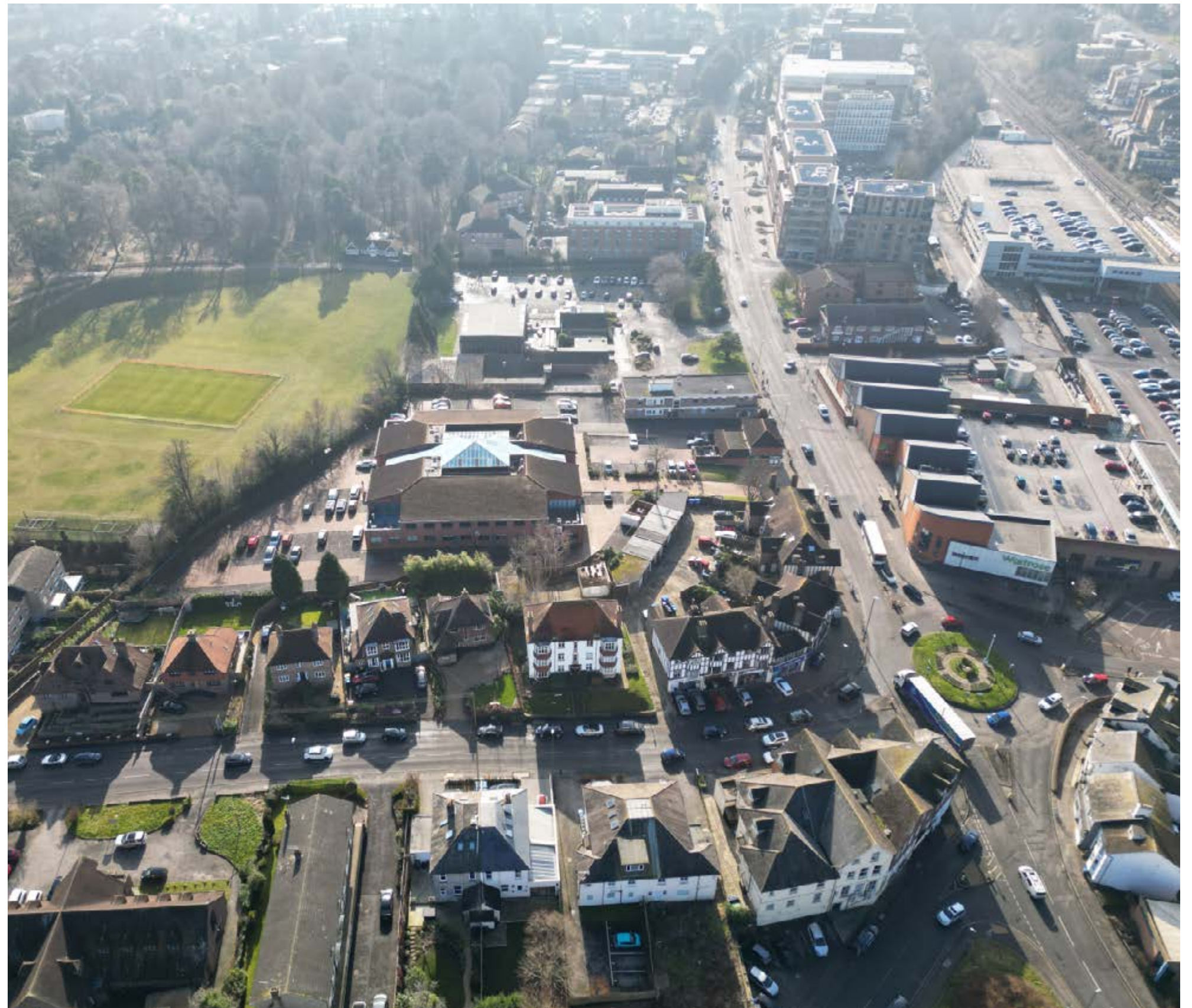
Aerial view across the site looking south along Perrymount Road. The difference in scale of buildings on the east and west sides of Perrymount Road can be seen clearly. The green fontage and tree line which currently starts from the Clair Hall site can also be seen on the east side of Perrymount Road.
