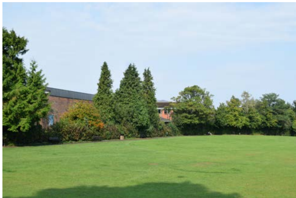
View point 6. Existing view. The roof of Sussex House is visible above the trees
