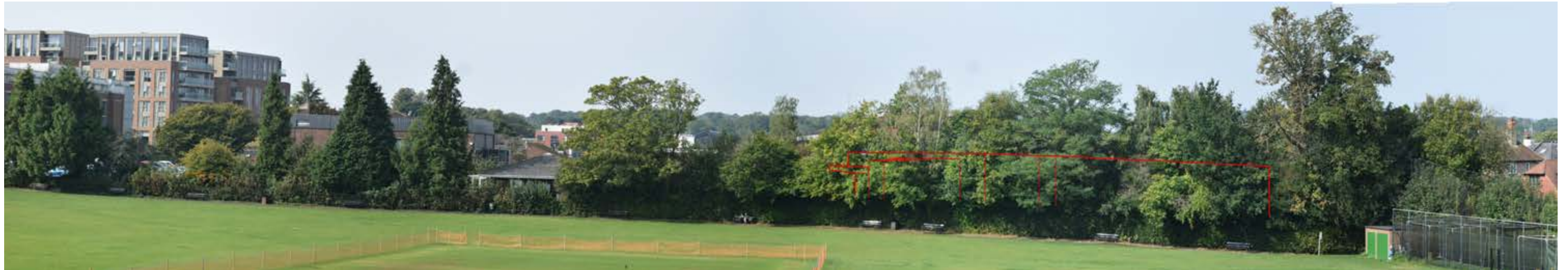
View point 1. Existing view, with the outline of the building shown in red. The building sits lower than the existing trees
