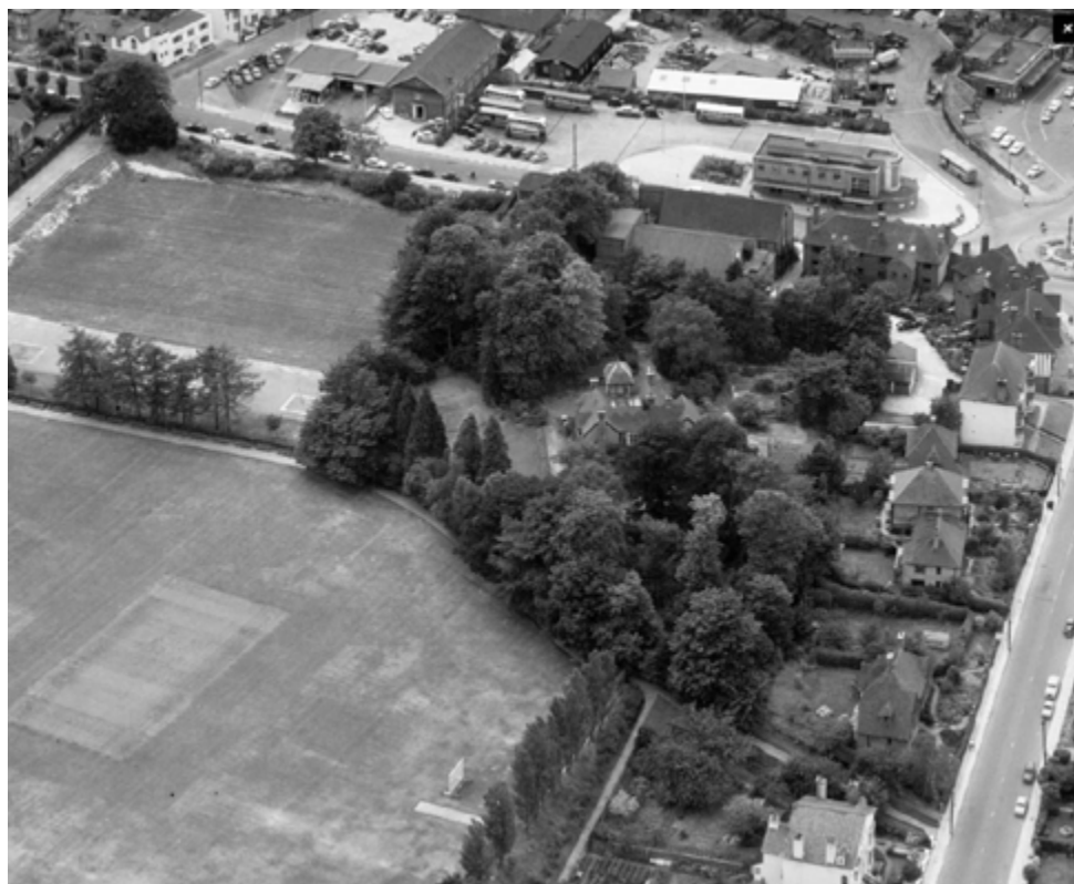
An extract of an oblique aerial photo of 1961. © Historic England EAW094356
