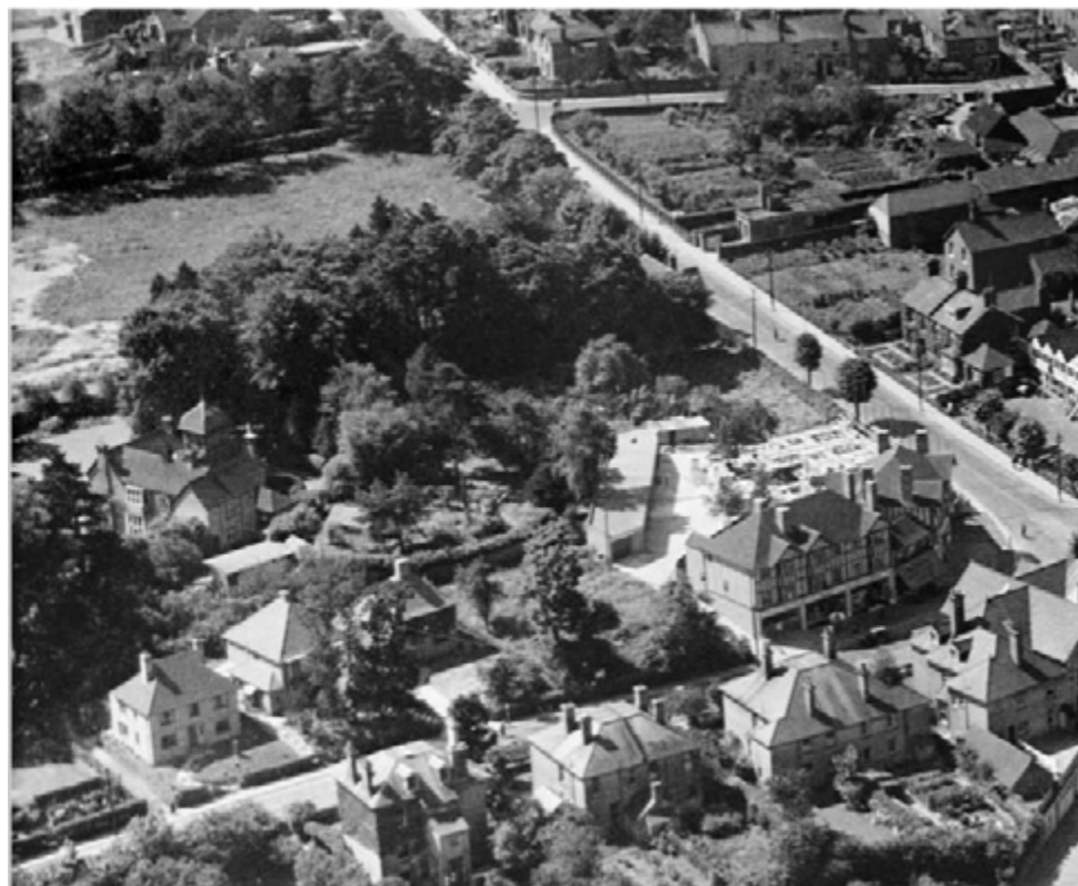
An extract of an oblique aerial photo of 1932 from the NE, of the site. © HES EPW039526
