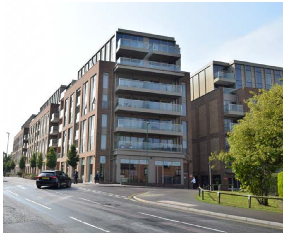
The Perrymount Apartments, Perrymount Road
