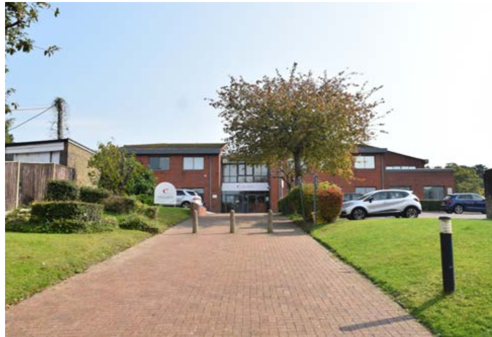
The view from Perrymount Road looking up the pedestrian access route to Sussex House. The trees along boundary with Clair Park and beyond can be glimpsed.
