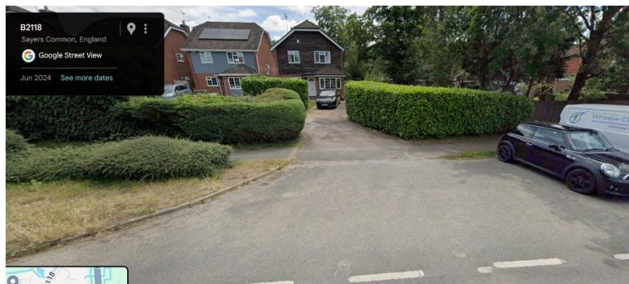
For the southern access the footway running across the driveway requires reconstruction and levels adjusted to make even. Kerbs could be provided across footway (dropped to accommodate tactile paving).
