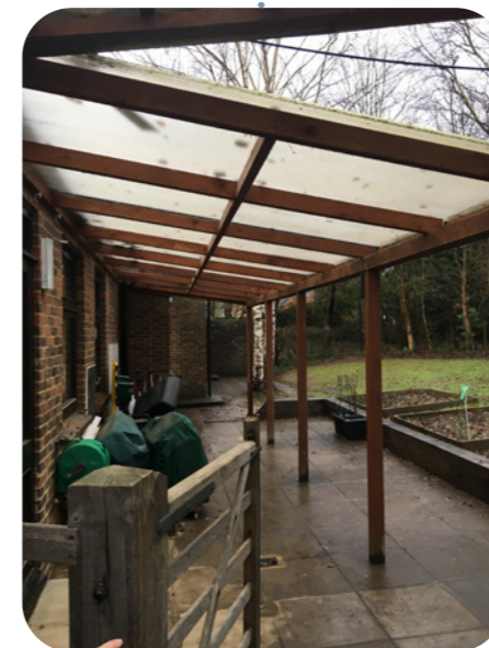
Existing Timber Canopy
