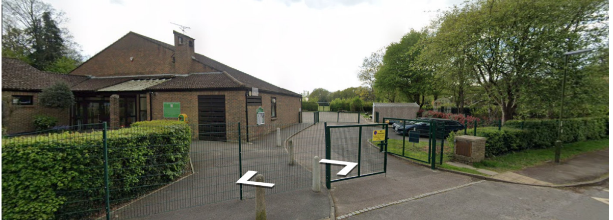
Figure 2: Access from Vicarage Lane
