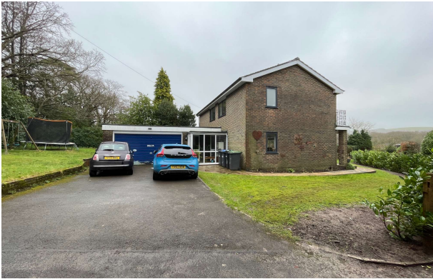
View from rear South Bank access road West Elevation
