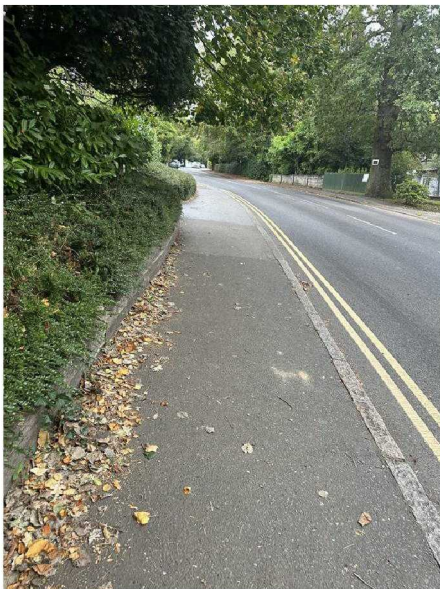
Photograph 5: Footway along Keymer Road
