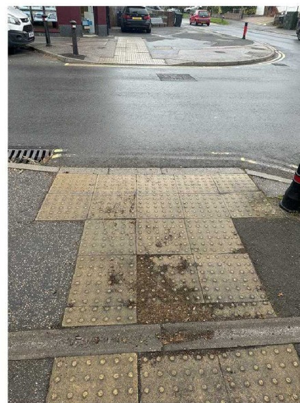
Photograph 6: Dropped kerbs and tactile paving towards amenities
