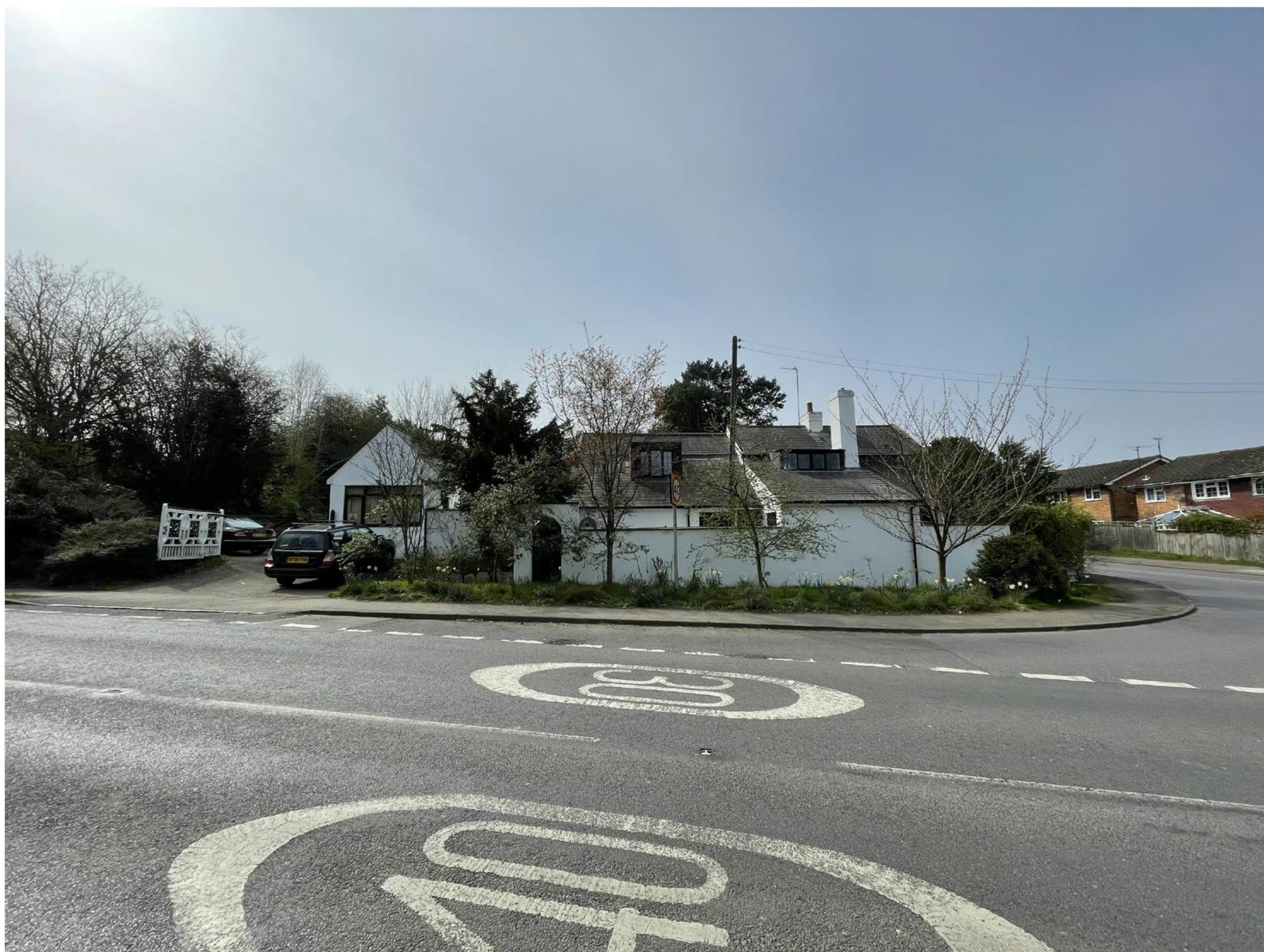
Plate 30 North-eastern façade of Greyfriars
