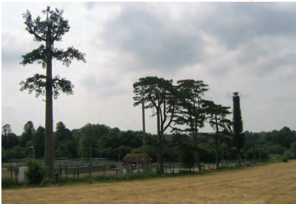
Disguised telecommunication masts near Cuckfield
