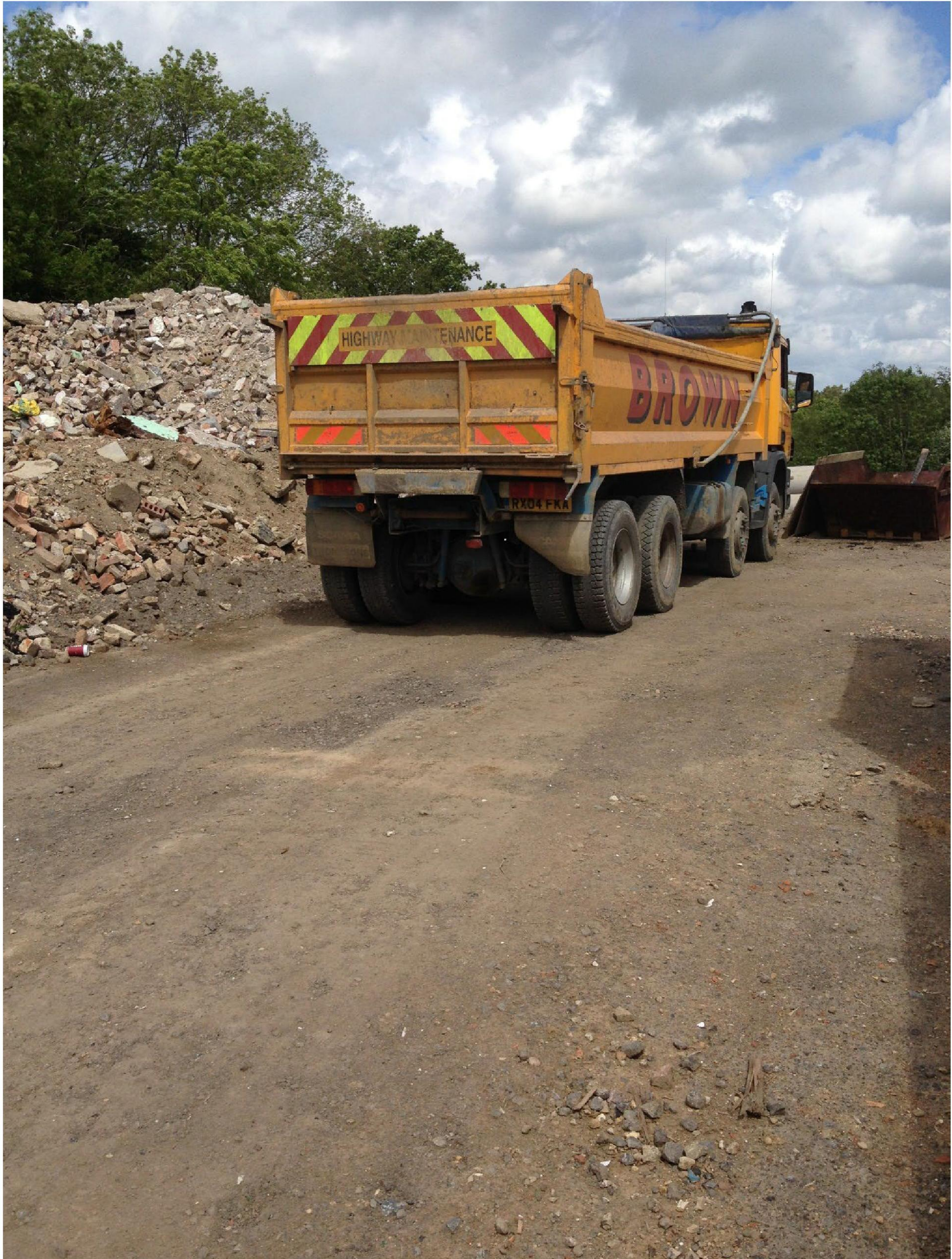
RX04FKA in Bolney compound next to large stockpile of material awaiting crushing.
