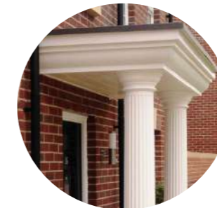
Entrance Canopy (painted white)
