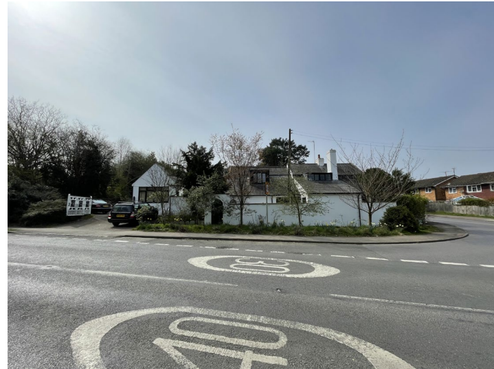
Plate 6 North-eastern façade of Greyfriars
