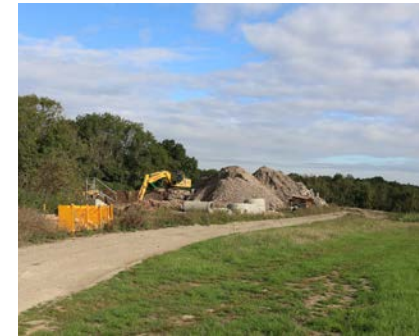
View looking north
