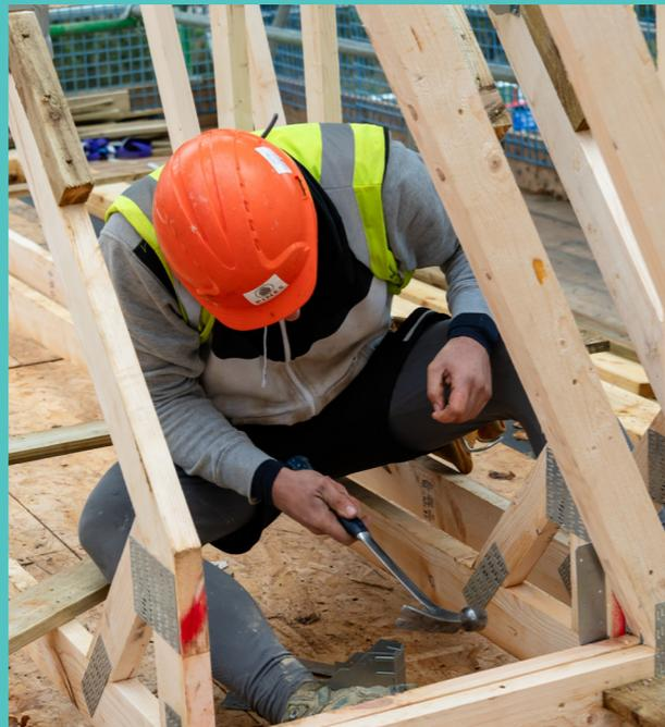
Image of Bellway's low carbon timber-framed homes being built at Brookleigh
