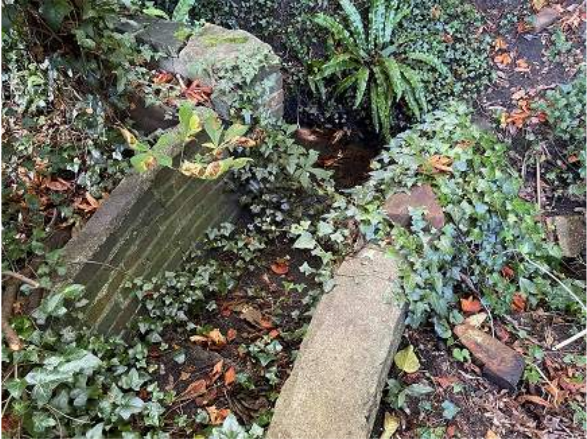
POSSIBLE SURFACE WATER OUTFALL INTO WATER COURSE
