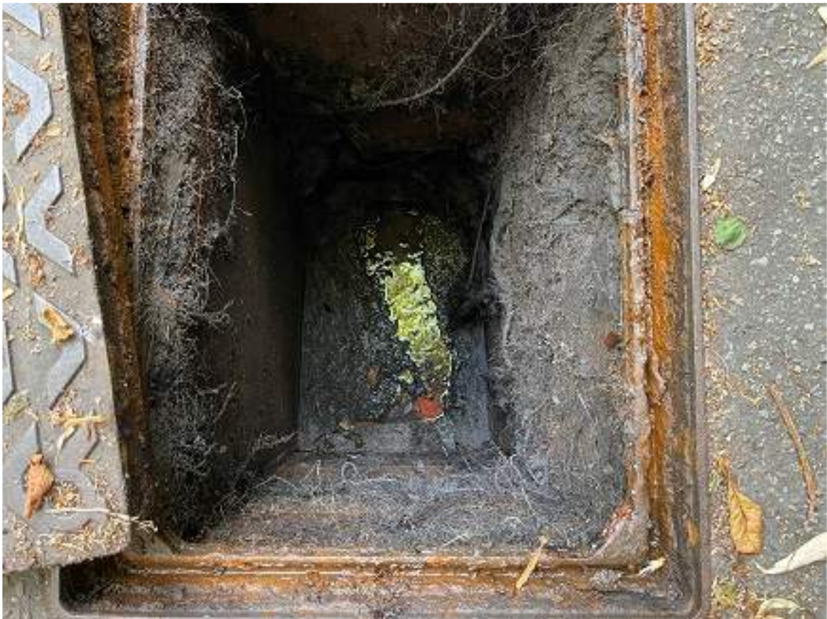
MANHOLE S1 (HIGHWAYS DRAIN)
