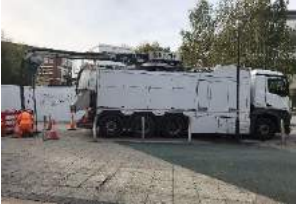
HIGH PRESSURE JETTING
